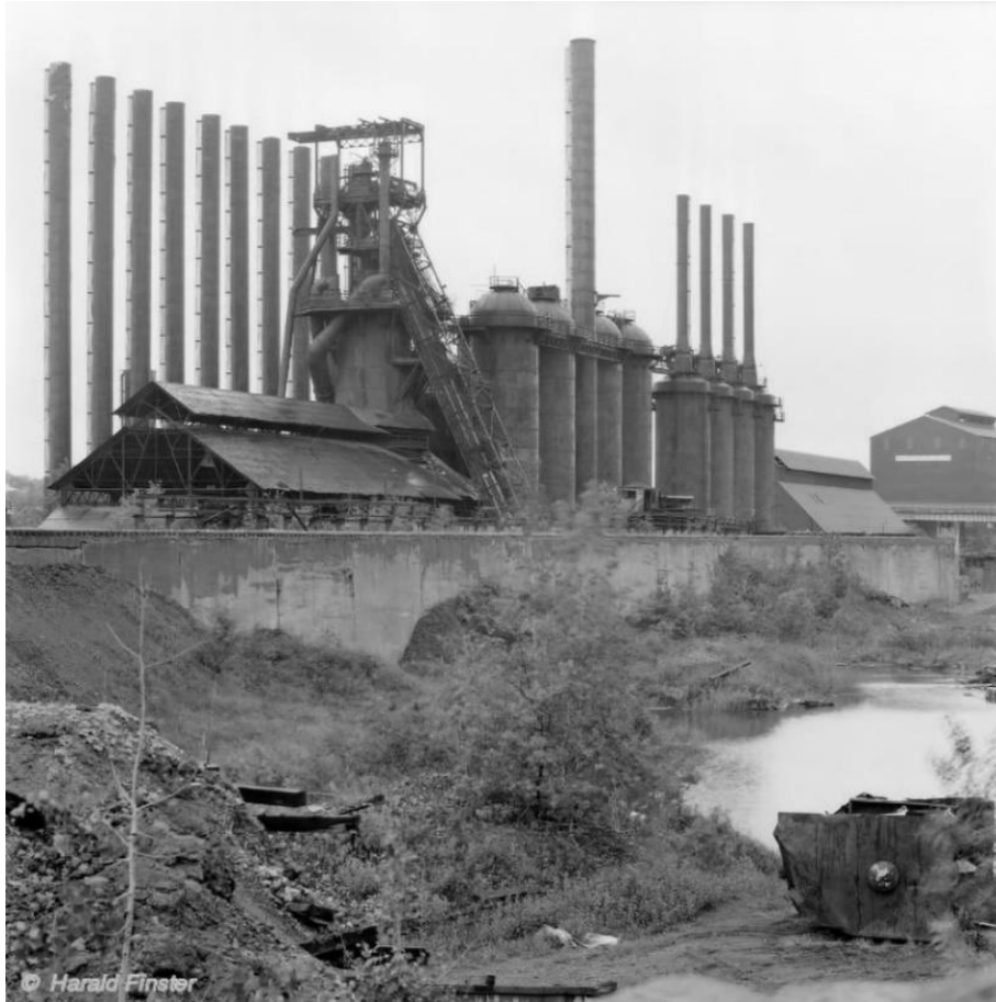
Image 10. Photo of the Jeannette blast furnace at the Brier Hill Works of the Youngstown Sheet and Tube Company, 1992. Photo by Harald Finster, used by permission.
