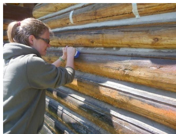
Figure 6. UW student Andrea Lewis cleans logs with abrasive brush after applying a cleaning solution. (Mary Humstone, 2011)
