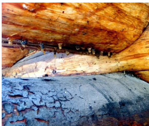
Figure 4. Black fungus growth on logs as a result of treatment with linseed oil. (Mary Humstone, 2011)
