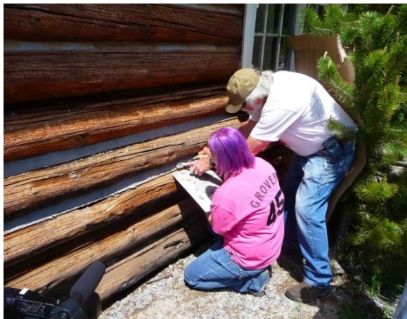
Figure 11. Harrison Goodall shows student Cassie Loveland how to apply daubing to the logs of the boathouse at AMK Ranch. (Mary Humstone, 2011)
