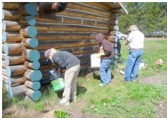
Figure 5. Team members prepare a log wall for testing to compare the effects of different log cleaning techniques. (Mary Humstone, 2011)
