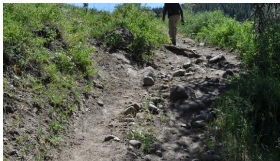
Figure 5. Buffalo River trail- showing damage from horse traffic. Trails widen, become deeper and lose topsoil near trail heads.
